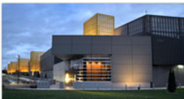
Raging Wire Virginia Campus
